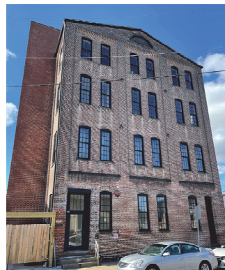
MEYERHOFF building , last used by Mrs. Smith's and vacant for years, was restored for $2 million by Rockwell Development.
